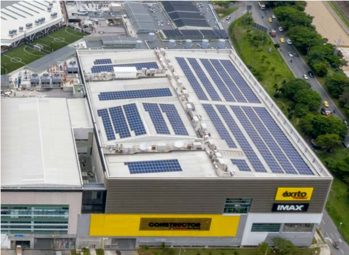
Viva Envigado has the fifth photovoltaic plant in the Company. It generates more than 451 kw/h with 2,700 m 2 of solar panels and supplies up to 20% of consumption in the common areas of the commercial complex during maximum sun radiation hours
